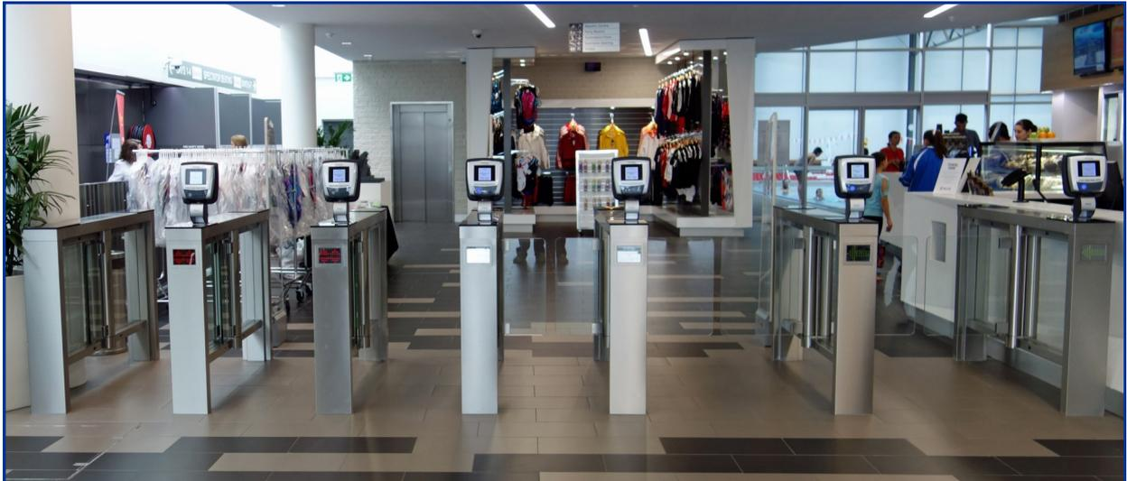
*'The EasyGate SG from Centaman Entrance Control integrated seamlessly with the Links Modular Solution POS system. Visitors scan their RFID or Bar Code cards at the Gantner readers and the gates open instantaneously.*
